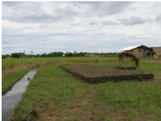
Figure 10: Backfilled foundation for aviary.
