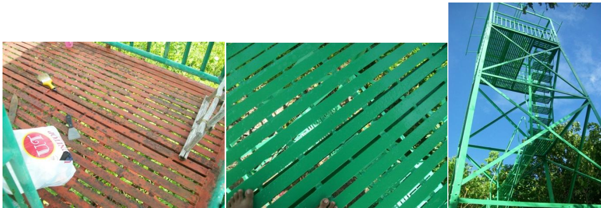
Figure 9. The left side picture shows the platform before it was repainted and the middle photo shows the same platform after removing rust and repainting was completed. The tower is ready for visiting guests and birders. ©KFI
